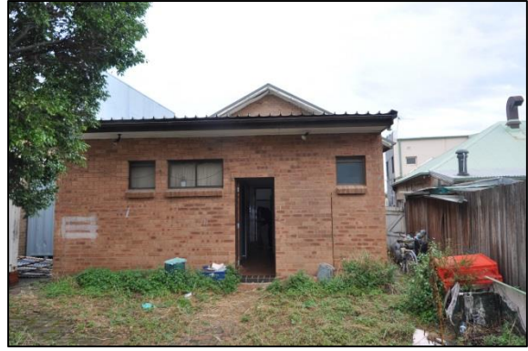
Figure 20. View of northern (rear façade) across the courtyard. Note the pitched roof of the original building and skillion roof of the extension.
