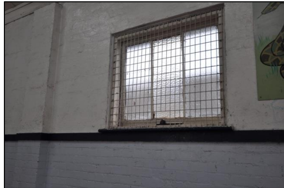
Figure 27. Example of original windows.
