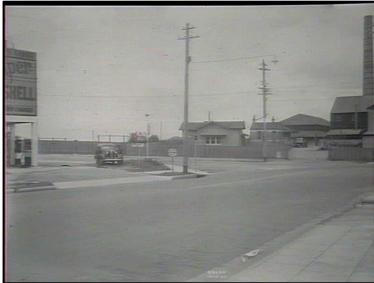
Figure 10. The Forest Rd and Durham Street intersection c. 1937. (Source: State Library NSW, http://www.acmssearch.sl.nsw.gov.au/search/itemDetailPaged.cgi?itemID=201639 , accessed August 2015.
