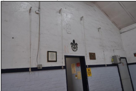
Figure 28. Scouting paraphernalia affixed to wall.
