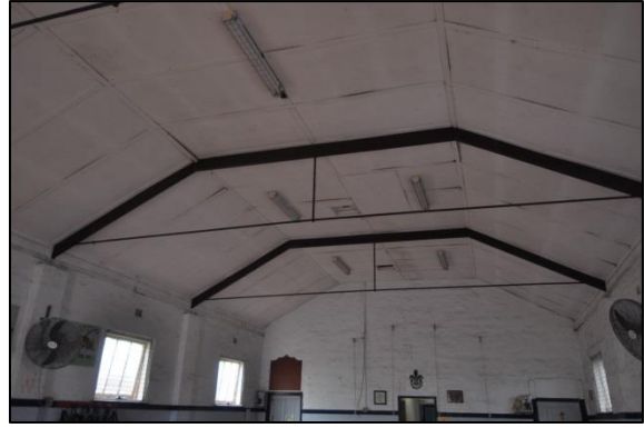
Figure 25. View of ceiling showing fibro panels, truss.
