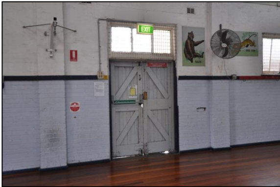
Figure 26. Example of original door.
